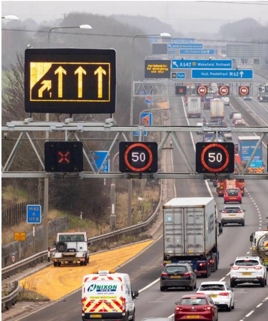
M62 junction 30 dynamic hard shoulder motorway
