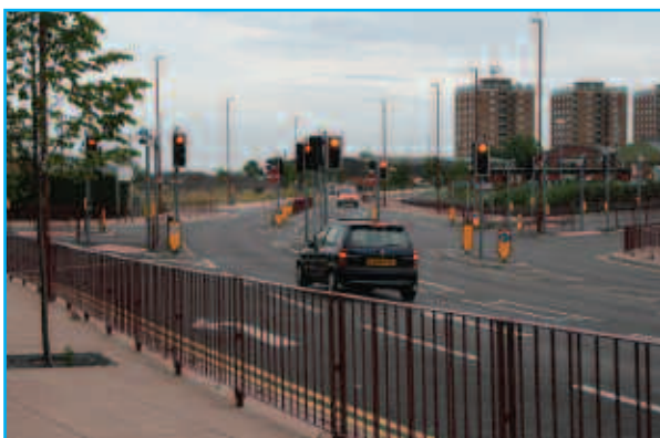
Newly-implemented highway scheme with extensive guardrailing
