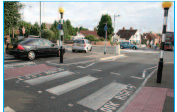
Zebra crossing located close to road junction.
