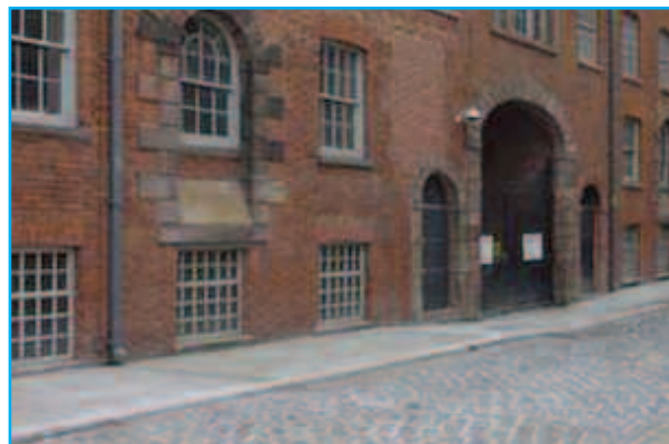
Access to commercial property with limited visibility.
