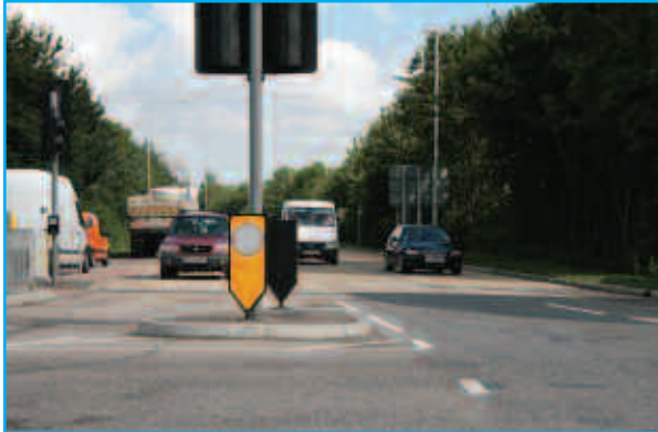
Keep left bollard, with rear face uncoloured
