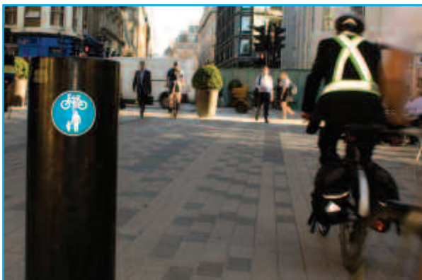
Sign mounted at low level
