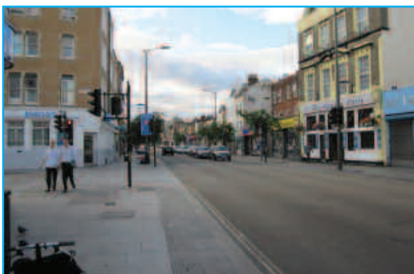
Raised table across side road at signalised crossing – Walworth Road MPR scheme.
