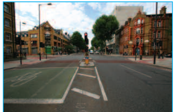
Traffic signal junction with clear and simple pedestrian crossings and advance cycle stop lines. Note lack of guardrailings and buildings close to junction corner, and tight corner radii.
