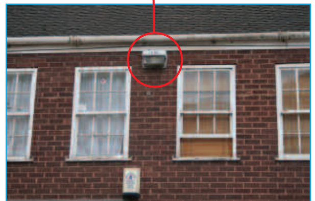
Inconspicuous lighting units on buildings help to minimise clutter in this village high street.
