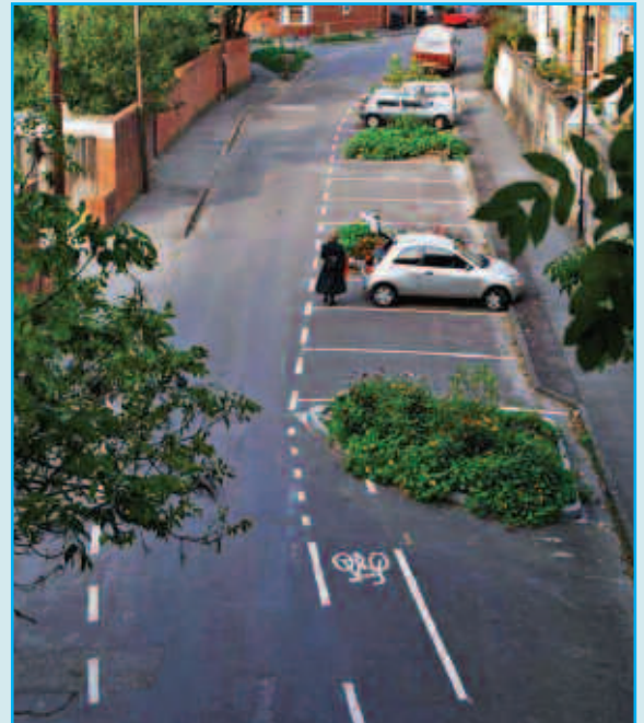
Mina Road, Bristol – After
