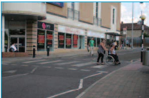
Zebra crossing on raised table.
