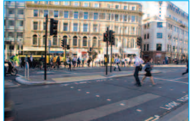
Staggered signalised crossing without guardrail
