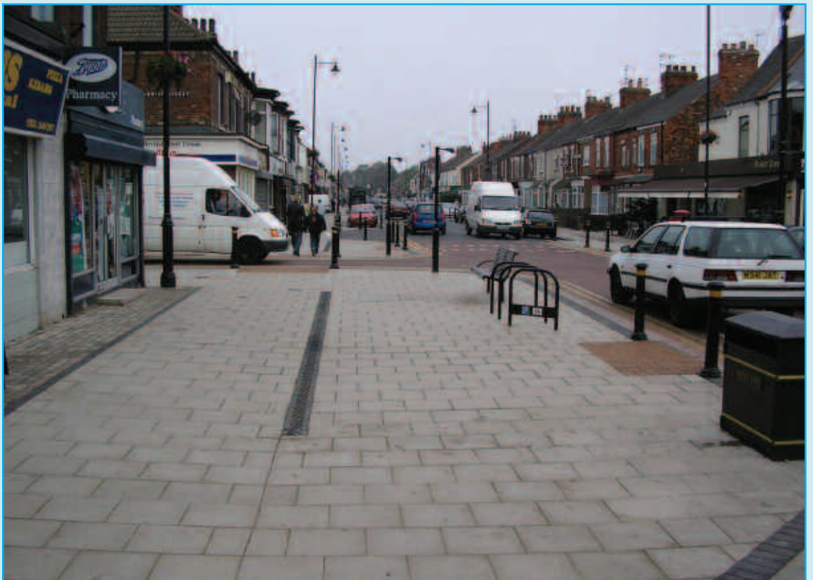
Footways widened significantly by narrowing carriageway
