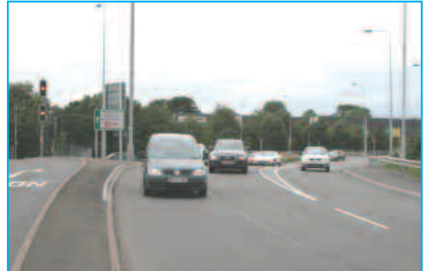
Cyclists leaving this roundabout can find themselves in the outside lane of a dual carriageway.
