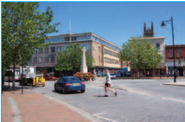
Roundabout in Taunton town centre with proceed left signs to Diagram 606 but no black and white chevrons to diagram 515. Note - cobble surface is difficult for cyclists.
