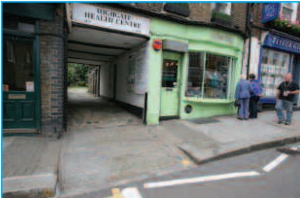
Footway crossover access to commercial premises
