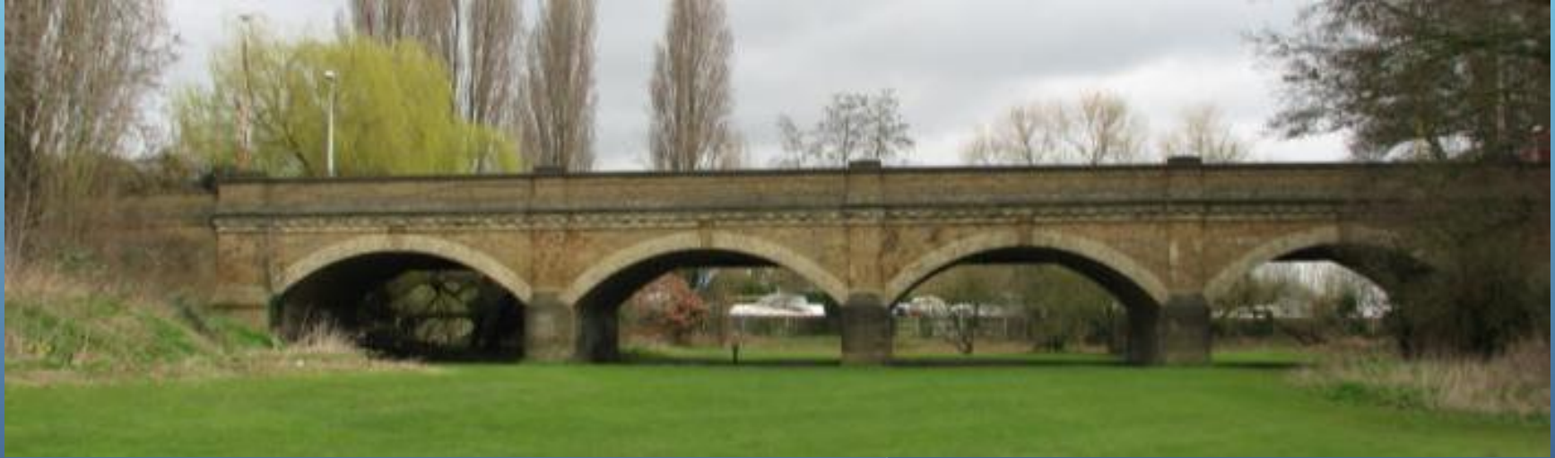
Cowey Sale Viaduct
