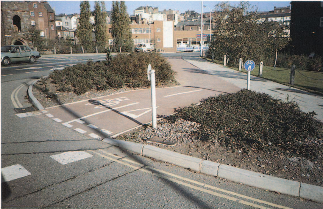
32: The use of red slurry seal clearly defines this section of the Exe Cycle Route. (Photo: Devon County Council)
