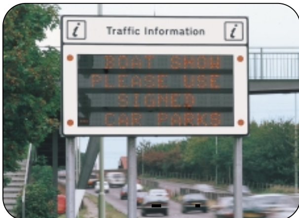
City information sign – here showing an advisory message to drivers approaching an event likely to cause significant queueing or congestion at peak times.
