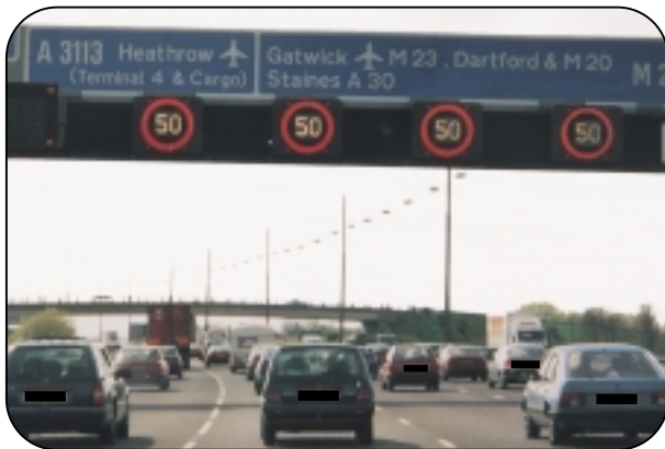
Lane control signs on the M25, showing enforceable speed limits under high-flow conditions.
